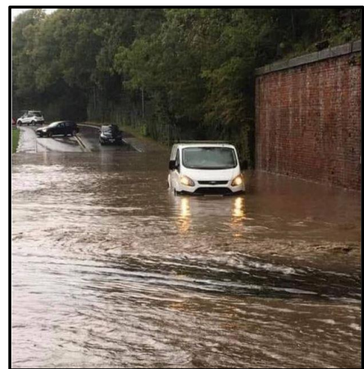
Photo 2. Low point junction of Church Hill
